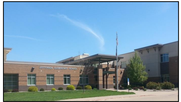
Jefferson Elementary – Renovated in 2011
